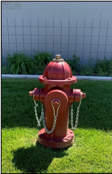
Photo 5-1: A typical dry-barrel hydrant with one steamer port and two 2 ½" ports.
