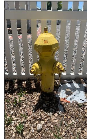
Photo 5-3: A typical Double 2½" with two 2½" ports.
