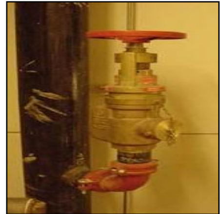
Photo 6-14: Adjustable Pressure Reducing Valve.
