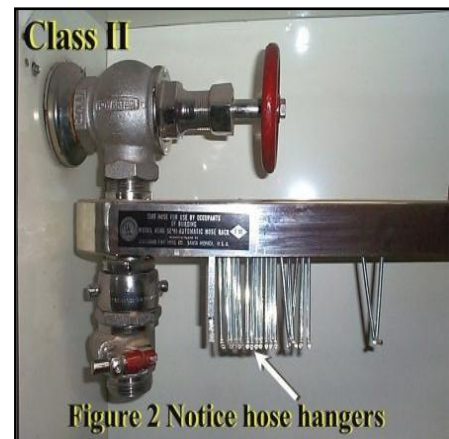
Photo: 6-2: A Class-II standpipe will have 1 ½" outlets and 1 ½" hose and is for occupant use.
