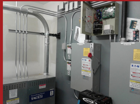
Mainline disconnect in elevator mechanical room
